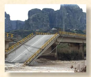
The collapse of the bridge was the result of harsh weather, heavy rainfall and flooding.
